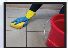
Grout Finishing
